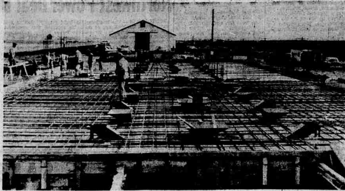
CONSTRUCTION OF THE $350,000 concrete grain storage elevator of the Winema Elevator Co., Tulelake, is well under way. The structure replaces the wooden elevator which burned to the ground last fall at a loss of $1 million. The burned building was filled to the brim with grain.
