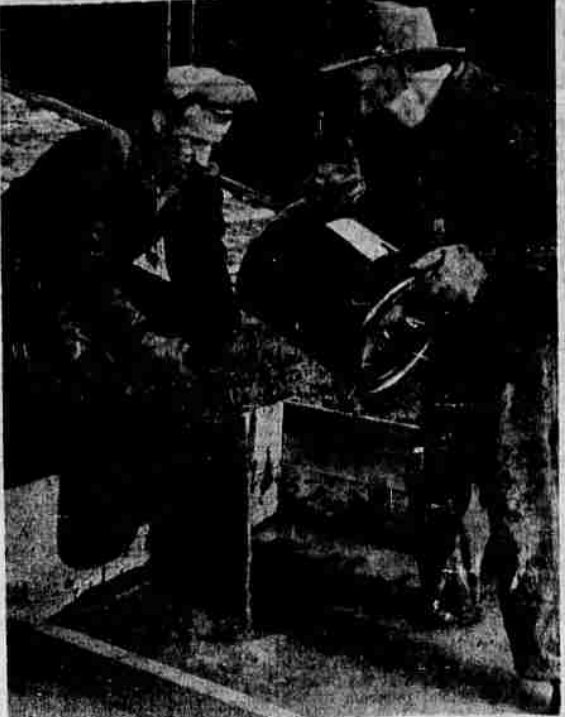
"A MAN HAS TO BE a mariner as well as a builder on this job!" is Russell Wilson's (right) sentiments as he answers a call to "Bail out!" by fellow worker, Norman Gale. The men ran into difficulty at the site of the new Klamath County Library and Museum building, when, following excavation, water began seeping in — to a depth of five feet in the elevator pit. To drain the water, men knocked a hole in the sewer line — just one of the unexpected that come up from time to time, and are brought under control. Could this be an assurance, though, that books in the county library won't be dry???
