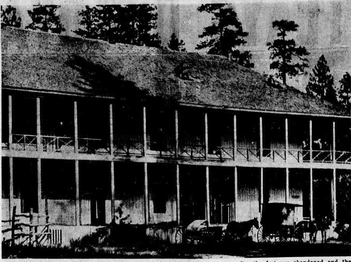
THE OLD OFFICERS QUARTERS at Fort Klamath had a gay look plus plenty of balcony space when the fort was fully staffed. This picture, brought in by Hal Ogle, was taken some time after the fort was abandoned and the old building had deteriorated badly.
