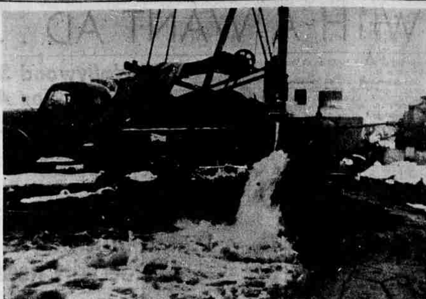
DRILLED BY PAT MCGINLEY. Tulelake, this well on the Buster Vaughn ranch, eight miles south of Silver Lake pumped 3500 gallons per minute when tested by Valley Pump and Equipment Co., Klamath Falls. The well, a 16 inch hole is 411 feet deep, but water rises to within 60 feet of the surface. Water from the well will be used for irrigation purposes.
