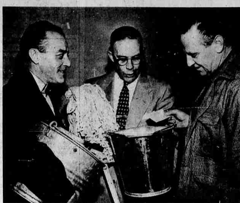
LEAKY ROOFS , which necessitated potted palms scattered throughout the room at the recent YMCA annual report meeting, have been taken care of by generous Lions. Check- ing the last drip is Brick Leach, right, with the check for $250 which took care of major roof repairs and made it possible for Paul Campbell, YMCA director, center, and L. Earn- est Taylor, Lions Club president, to put away the mops and pails. Campbell says, though, that they intend to hang on to them for another rainy day!
