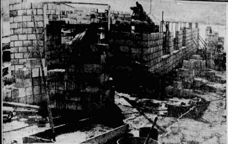
WINTERTIME CONSTRUCTION was underway at the Monroe Boat Docks when the Herald and News photographer took this picture of a new pumice brick showroom, storehouse and the Yacht Club.
