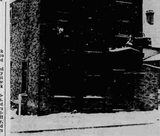
ROARING FLAMES SWEEPED through a Klamath avenue rooming house Sunday morning imperiling the lives of nine tenants and destroying the two-story building. Pictured (upper left) Leslie Bleakman, Arthur Gate and Matt Pollari who leaped from second story windows. (Center) — Fire Chief Roy Rowe examining the ruins. (Right) — Building enveloped in smoke and flames. Bottom, the structure after the fire was extinguished.
