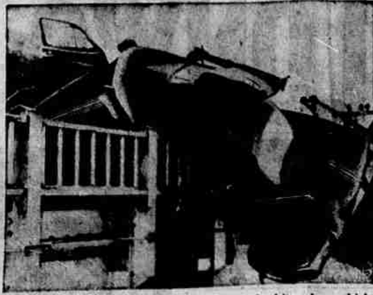
DEER BAGS HUMAN—Split seconds after he hit a deer which was crossing the highway near Salt Lake City, Utah, Jesse James Scott, father of two children, died in this mess of twisted steel which was once a new car, as it smashed, out of control, into this bridge railing.
