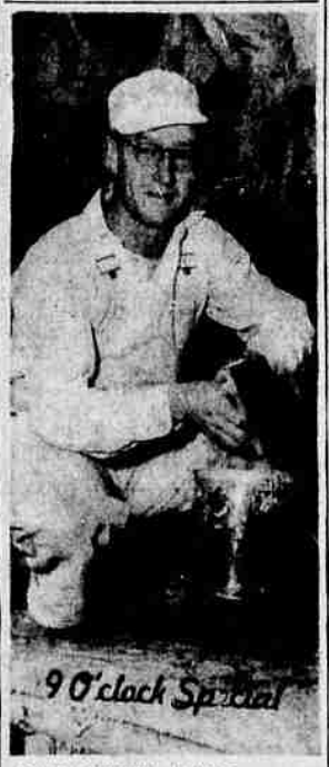
M. E. FISHER, 1842 Summers Lane, employed by the K. C. Painting Co., was starting the morning's work when the Nine O'Clock cameraman stopped by. He and the K. C. crew were painting the Klam- ath Temple at Eleventh and Pine.
