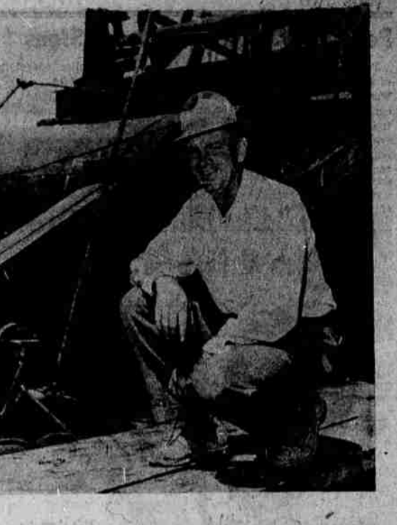
"WE PROVED IT COULD BE DONE," said Ed Duckett, Tulelake, city water commissioner at the site of the city's deepened well, this week as preparations were being made for drilling a second well near the present one. The deepened well, now over 2700 feet deep, has given the city its first palatable, soft water for domestic use. The N. C. Janssen Drilling Co., that recently completed the deepening program will drill the second one.
