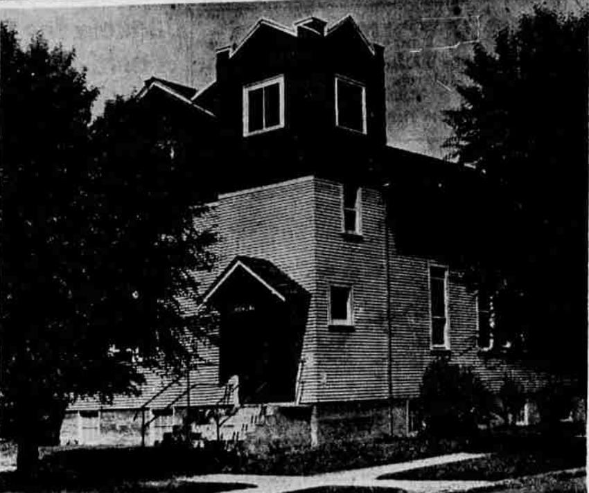
THE CHURCH OF THE NAZARENE was just a hole in the ground during depression days. This present structure has since been completed and stands at the corner of Garden and Martin Streets.
