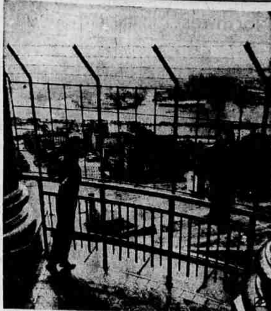
FENCING WITH SUICIDE — Addition to fence enclosing walk atop Hamburg's famous church spire, "Michel," is designed to prevent suicides from jumping from 433-foot tower.
