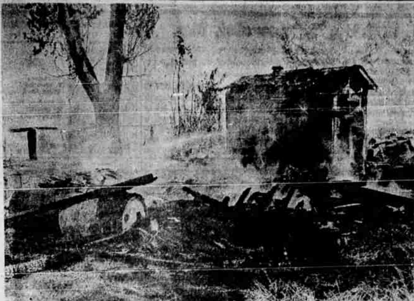
A MAINTENANCE BUILDING at Henley School was destroyed by fire Friday. Above, members of the County Fire Department douse the still burning timbers.
