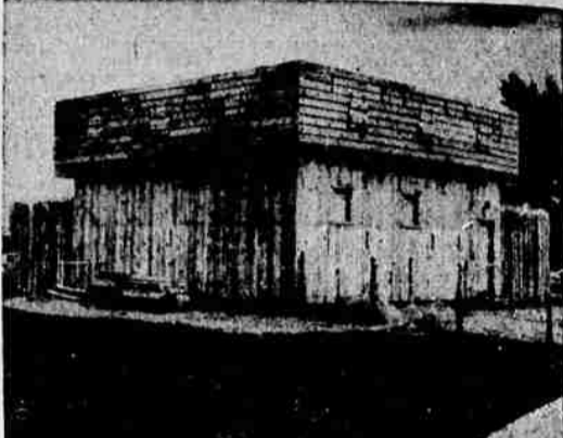
PILGRIMS STILL PROGRESSING—This authentic, full-sized reproduction of the Pilgrims' first meeting house has been erected at Plymouth, Mass., near historic Plymouth Rock. It is the second major project to be undertaken in building "Plymouth Plantation," a memorial to the early settlers. No nails were used. Historically authentic "trunnels"—wooden pegs—hold the structure together.
