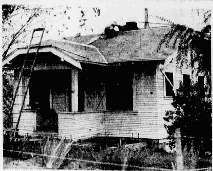
A NEW ROOF is being put on for Mrs. Viola Heath, 937 California. An A. E. Bailey worker was working around the chimney when this picture was snapped.
