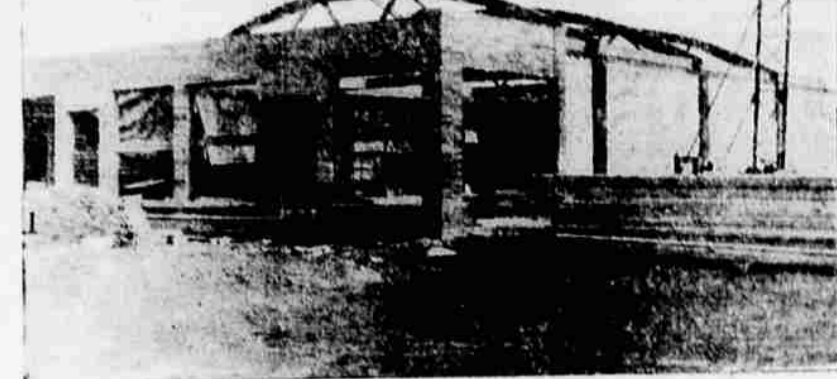
THIS NEW STRUCTURE, an addition to the Suburban Drug Co., South Sixth Street will be ready for occupancy in early fall. The tile and Roman brick building is being readied for a general merchandise, self-service setup with large paved parking space. Co-owners of the Suburban Drug are Robert Waggoner and Allen M. Urban. This is the second addition to the building in the past year.
