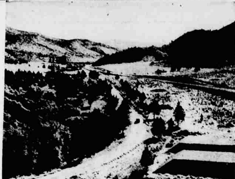
OLD KINKS IRONED OUT. The Jones Ranch-Mitchell paving job in Eastern Oregon on the Ochoco highway, 22 feet wide, estimated to cost about $821,000, is scheduled for completion August 31, 1953. Old road is in the foreground. The new cuts curvature from a total of 1621 degrees to 404 degrees and will save both time and gasoline.
