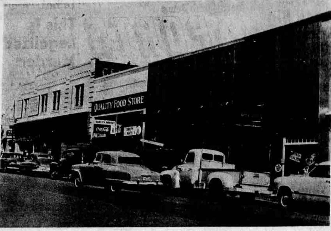
MAIN STREET GETS NEW LOOK this spring as more and more store fronts are worked over. This photo shows the work currently being done on the Main street block between 8th and 9th.
