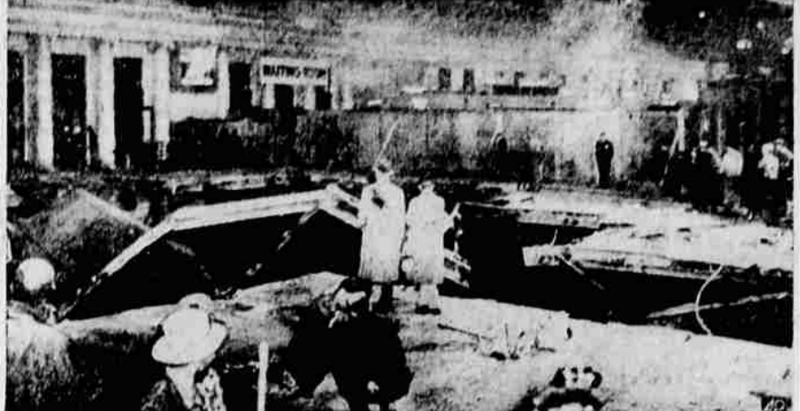
CONCOURSE WILL NEED PATCH—Most of the runaway train has been removed, leaving a big, jagged hole in the floor of the Union station, Washington, concourse at workmen go about the business of making it fit for use again. The locomotive (left) will be dismantled and removed on the lower level. Partitions (right rear) have been put up to separate the damaged area. The train dropped through the concourse floor just short of the waiting room.
