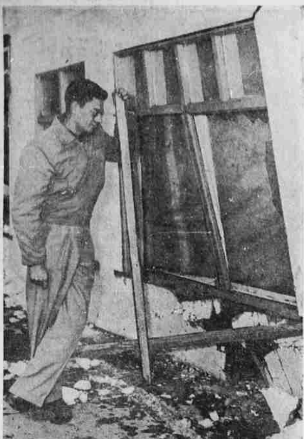
A CAR THAT WENT OUT of control on East Main Street across from Mills School pushed in the front of this building owned by Jack Nolan and occupied by Oregon State Highway Department. Here — W. H. Officer, draftsman for the department looks over the damage. The car was driven by Melvin Oliver Olds, 27, who was fined $50 in municipal court for reckless driving.
