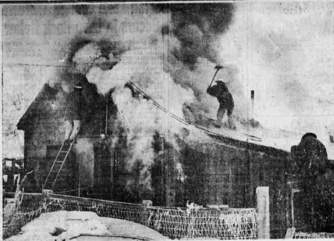
A FIRE BREAKING OUT in an inside wall Monday virtually destroyed this small house at 720 Front Street, leaving homeless Mr. and Mrs. Marshall Moon and their four small children.
