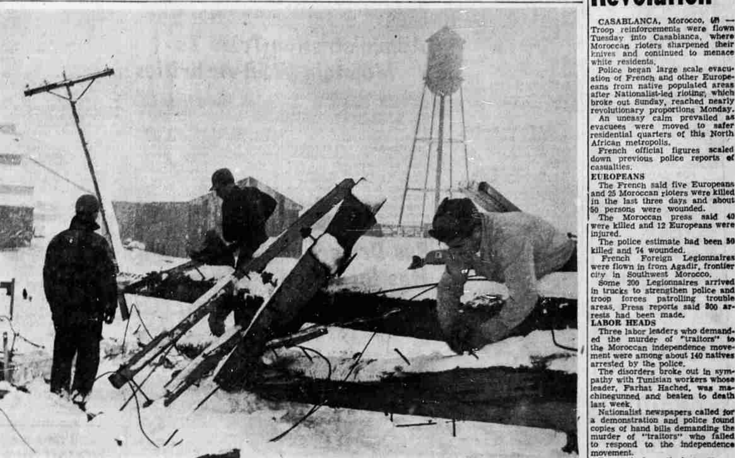
ONE OF THE CAUSES of Klamath Falls' electrical troubles during the current storm was this tangle of downed power poles and lines near Klamath Basin Pine Mills South of town, which dumped the power line into the Klamath River. Here Copco workers attack the wreckage in their effort to get the power situation back to normal.
