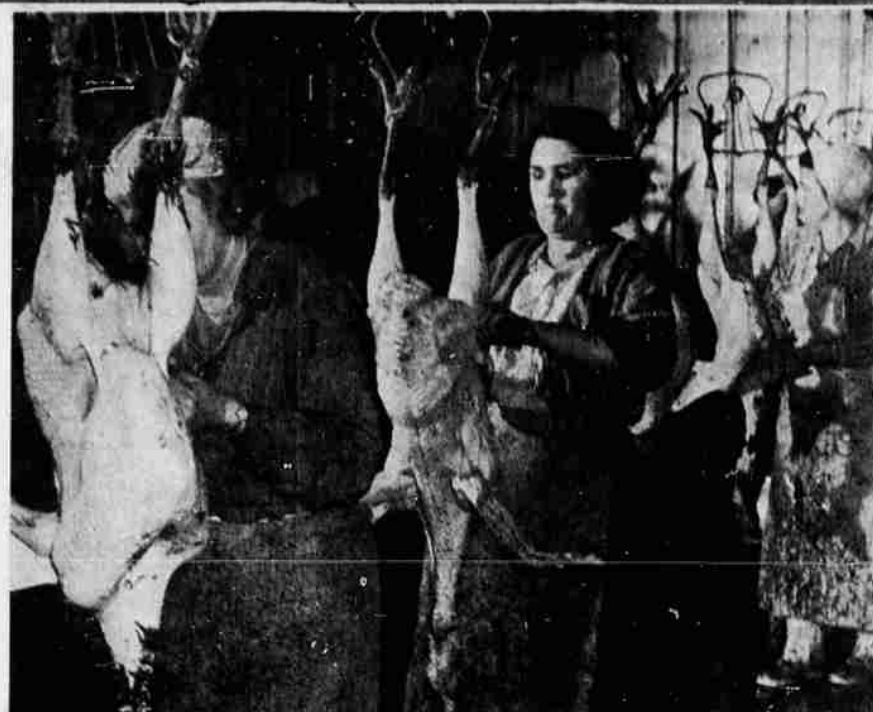
PINNERS follow turkey chain from de-feathering machine, taking pin feathers from the flesh. Turkeys take from 10 to 15 minutes each to get through line, but 15 or 20 birds are being worked on all the time. About a turkey every 45 seconds comes off this mass production.
