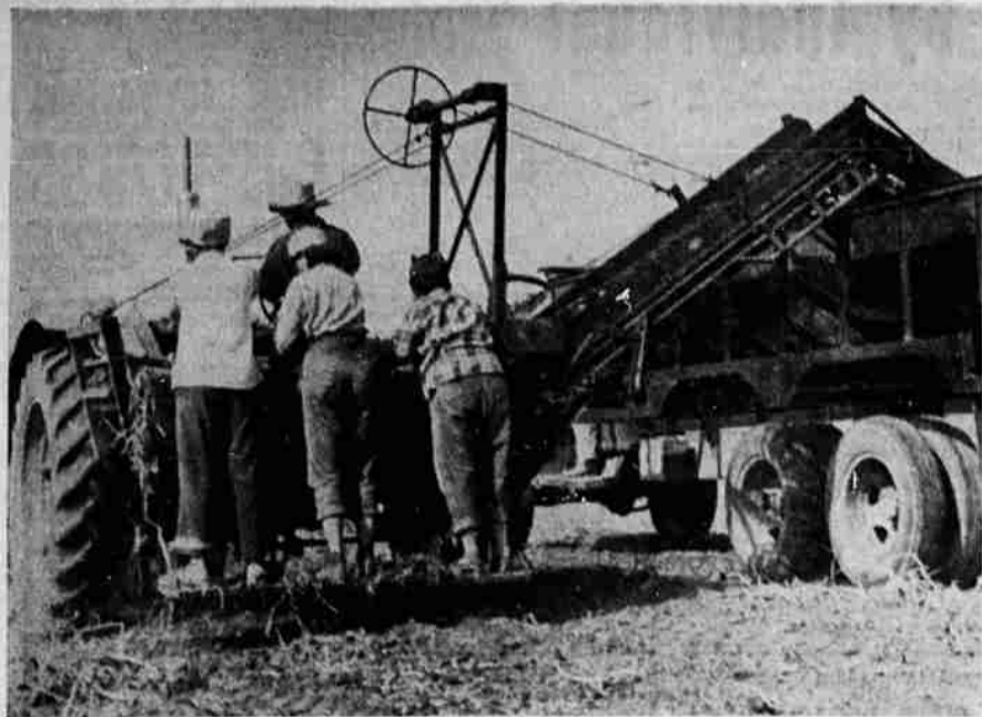
THIS IS A Lewis Manufacturing Co. rig being used on the G. P. Wu place near Bonanza. It takes seven persons and the machine here to do the work of about 25 to 30 pickers and cellar-men under the conventional picking system.
