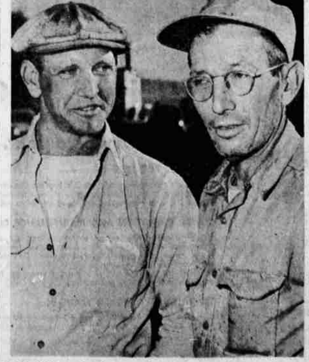
TOP GUYS, roofers that is, make today's special. Above (l to r) are Doyle Allison, 445 Market Street, and Jim Krans, Cozy Hotel, employees of the All-Type Roofing Company. They were working on the Lowell's Lockers building, 807 Pine Street, this morning.
