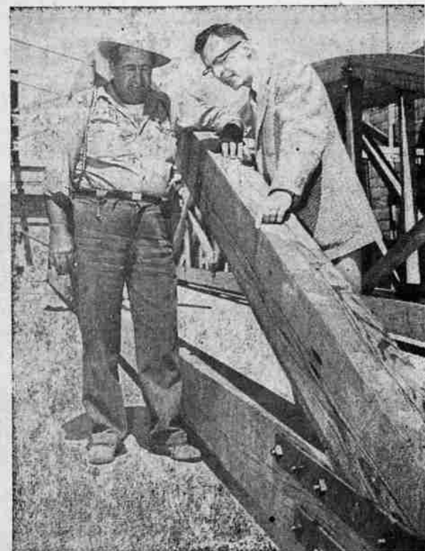
WEYERHAUSER TIMBER COMPANY'S structural trusses were used recently on two buildings for the first time in the Klamath Falls area. The buildings were the new homes of Klamath Bowling Association and the Hitchcock-Mosher Company. Above, installation of one of the prefabricated trusses is inspected by (left) Howard A. Burkhard, contractor, and (right) Wendell L. Huettel, assistant sales manager of Weyerhaeuser's Klamath branch.
