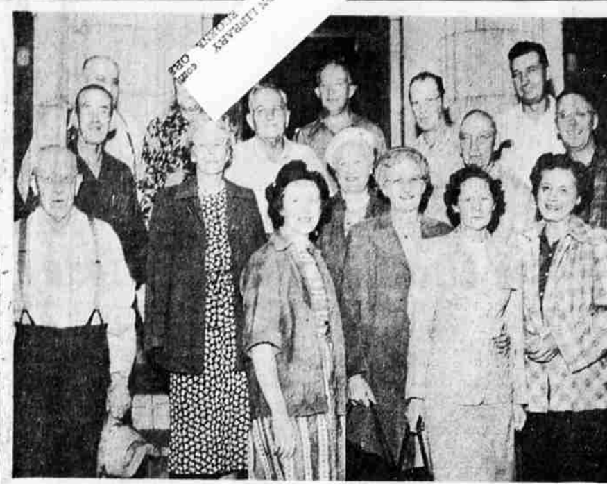
A TRIP TO TOKETE FALLS, where The California-Oregon Power Company is putting in several new power installations was made today by this group of local officials and civic leaders. The group was to spend a large portion of the day tramping over the Copco layout to get acquainted with what the company is doing to make more power available for its customers in this area.
