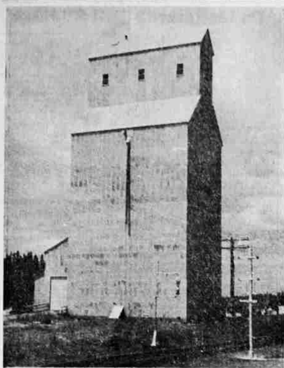
OUTSTANDING LANDMARK in Chiloquin is the Williamson River Farms grain elevator, beginning its second season in operation. The 127-foot structure was constructed by the Hensel-Liskey Tulana corporation. It has a capacity of 91,000 bushels of grain.
