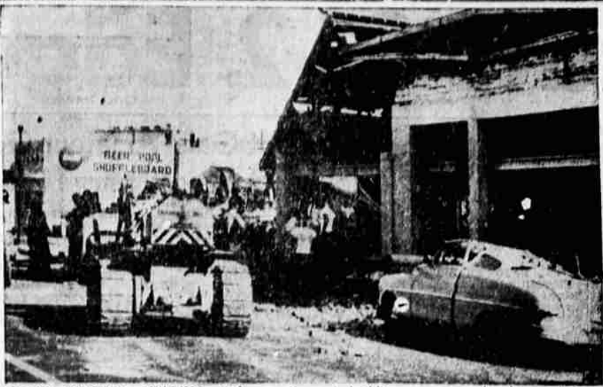
QUAKE WRECKED BUILDING —A farm equipment building was severely damaged in a violent earthquake which struck this mid valley city of 50,000 people. At right is an automobile which was damaged by falling bricks. The Bakersfield quake occurred Friday.
