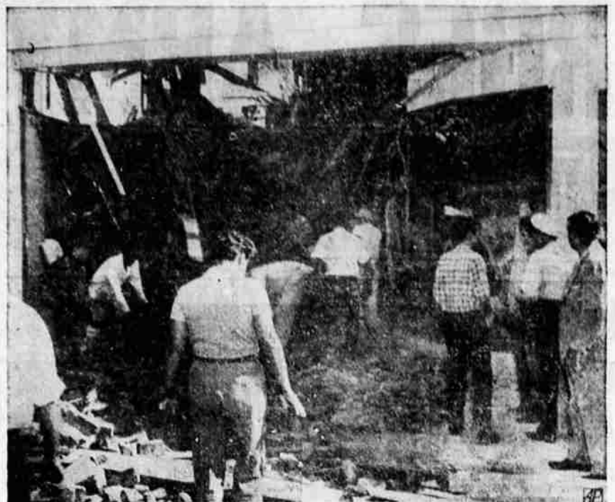
SEARCH FOR QUAKE VICTIMS —Volunteer rescue workers search through the rubble at the entrance to Lerner's store minutes after a woman victim of the earthquake which hit Bakersfield, Calif., had been removed from the debris. First reports showed two dead and many injured. Unofficial estimates placed damage in millions of dollars.
