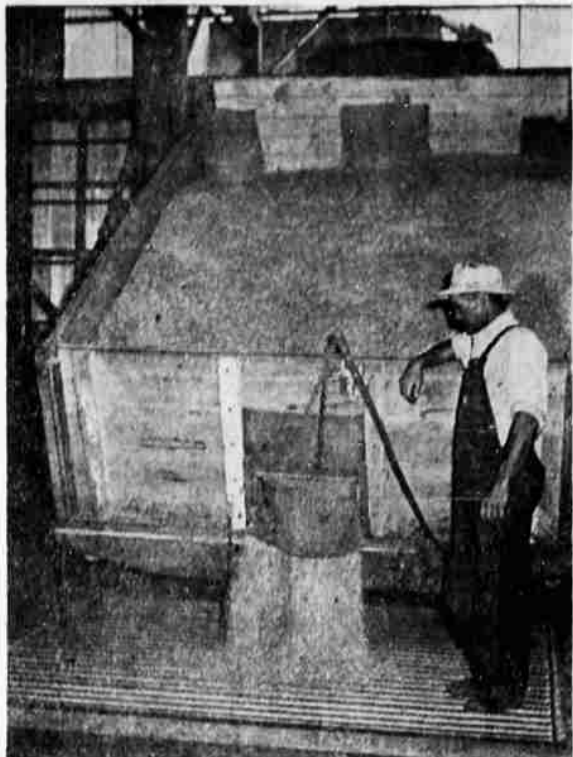
70 TONS PER HOUR capacity is what the new Pacific Supply Co-op grain bin takes. Here Paul Copen unloads some Karl Dehlinger oats which weighed at 4 1/4 pounds. The Co-op's new elevator is one of the tallest buildings in Klamath Falls, rising 106 feet above the street.
