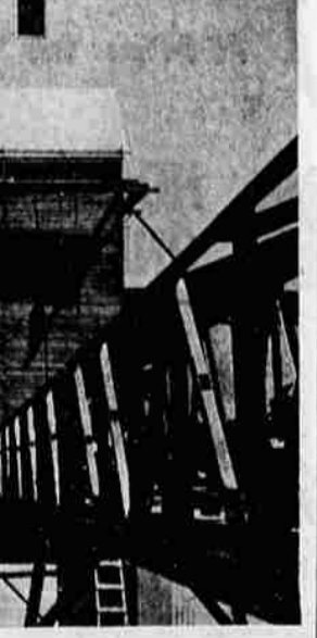
TALLEST?—The new Pacific Supply Co-op elevator, S. 6th and Spring Streets, may be the new tower in Klamath buildings. It rises 106 feet above the street level. The picture above was snapped from the catwalk which carries grain and other produce from the elevator to the railroad loading chutes.
