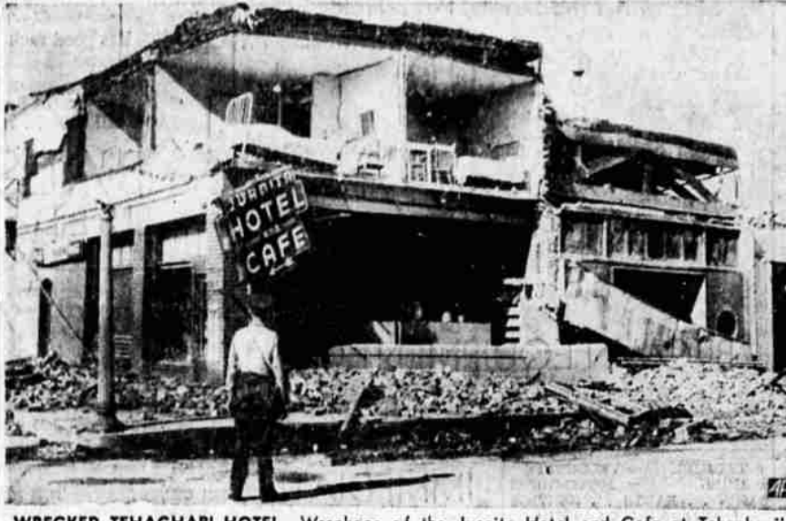
WRECKED TEHACHAPI HOTEL—Wreckage of the Juanita Hotel and Cafe at Tehachapi's main intersection after recent earthquake in Southern California interior, second most severe in the last half century. At least one victim was found in this hotel, as searchers still comb the wreckage.
