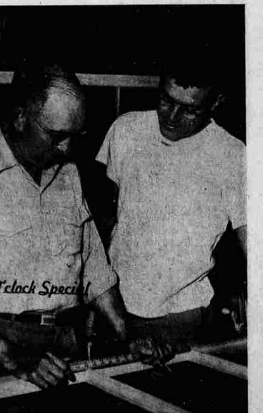
SNAPPED HARD AT WORK this morning were E. S. Robinson (left) of the Klamath Mill Work and Supply Co. and Forest Cullen, 2249 White Street. The men are pondering the details of a new window frame.
