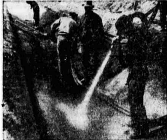
SHOTCRETE, a concrete mixture blown on with air pressure provides a smooth floor in the canals.
