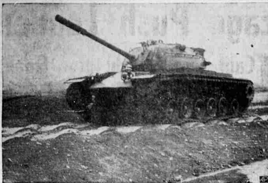
NEW MEDIUM TANK —Speeding over a "Washboard" course, the Army runs its new medium tank, the "Patton 48," through tests at Newark, Del. It has a lower silhouette than another U.S. comparable tank; has an egg-shaped, sloping elliptical hull and turret making it harder to damage with enemy shellfire; has wider treads; 90-millimeter, high velocity gun with quick change tube; external machine gun is controlled and loaded from inside.
