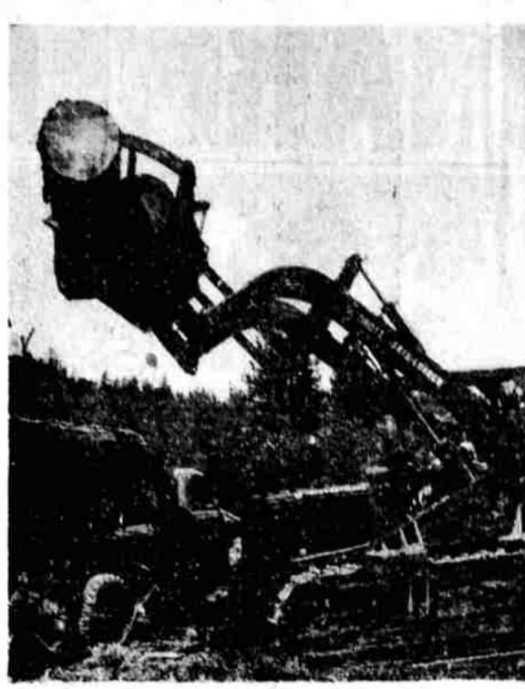
NEW METHODS of log loading were shown a group of foresters recently when the group toured the Adams Logging company, Paisley, woods operation. The skid loader is comparatively new in the west, only three being in use in this area at the present time; two with Adams and one used by Lake county. The rig enables operators to work in almost any terrain where trucks can be brought to the scene of logging.
