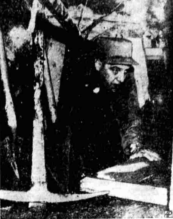
MAJ. DAVE KORN OF RICHMOND, VA., emerges through the opening of secret tunnel found in prisoner of war compound 76 Kojie Island after the compound was cleared of POWs in a bloody fight. At left are picks and shovels used by the prisoners. The tunnel was shored with planks.
