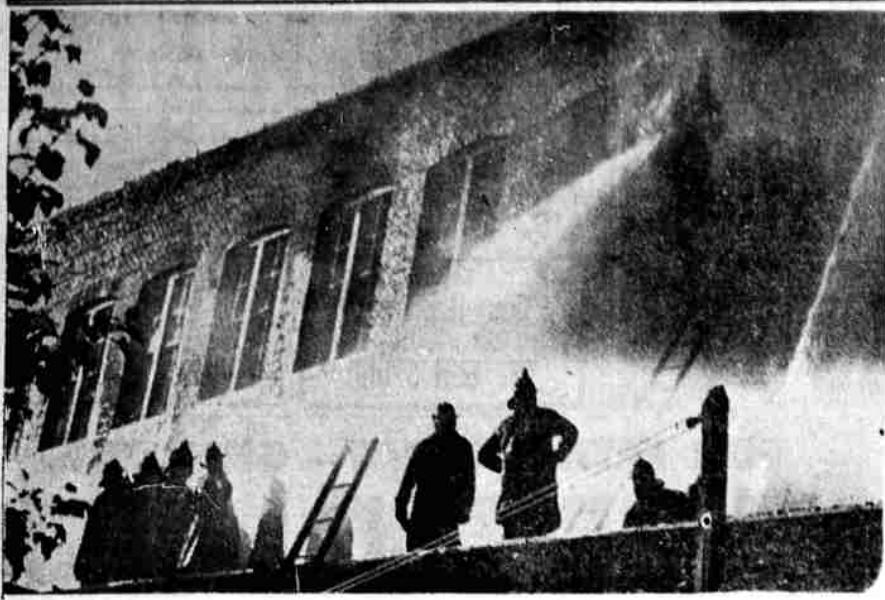
WITHOUT WARNING —Firemen atop adjacent building pour water on the blazing Terre Fiber Box factory in Chicago just moments before this brick wall collapsed on them. At least 12 firemen were injured. The victims were treated for injuries which included broken legs and arms and skull injuries. Fire damage was estimated at $200,000.
