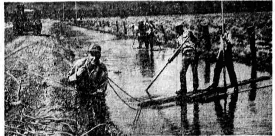
TOTE THAT BARGE—California Oregon Power Company linemen turned amphibious Friday while converting power lines in the Olene-Dairy area from 4,000 to 11,000 volts. Dragging a makeshift raft to dry land is Copco employee C. V. Childers of Klamath Falls, and on the raft are Paul Pettinger and Ed Furber. Further down the flooded borrow pit along the Lakeview highway are three unidentified Copco workers paddling upstream.
