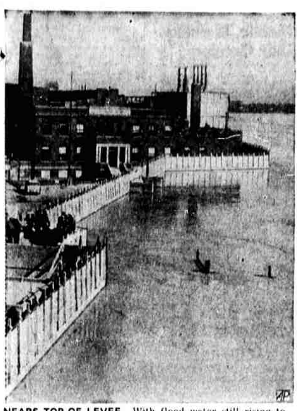
NEARS TOP OF LEVEE —With flood water still rising today, there's not too much space left to the top of the dike along the Missouri River. Wooden flashing atop the dike is an emergency measure placed on levee in hopes of containing flood waters should they go that high. In background, left, is the American Smelting & Refining Co., which stands well below the present water level.
