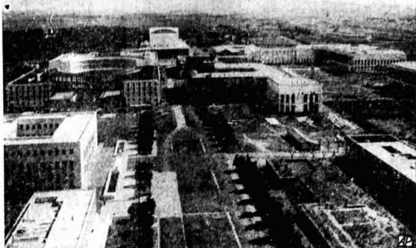
FAIR PROJECT RESUMES — After a start in 1937, the war and its aftermath, work again is resumed on these buildings to house an international exposition in Rome, Italy.
