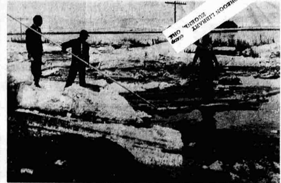
PLENTY OF ICE was in evidence at Thomas Creek, just west of Lakeview, when these pictures were taken Saturday morning. Picture at the top shows a crew picking ice out of a jam near the highway and shunting it down the canal. The picture at the right was taken at the same spot and shows a dynamite blast being touched off to break up the heavy formation. No serious floods have been reported to date but fears are held that rain may bring trouble.
