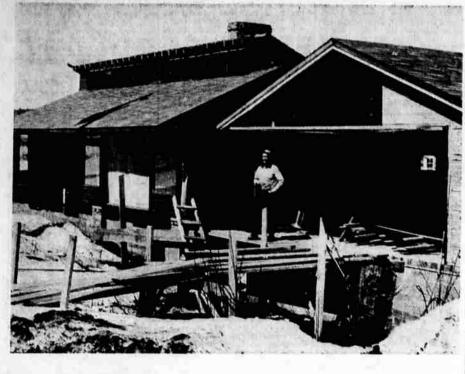
THIS NEW HOUSE, going up on Lakeshore Drive, is being built for Melvin McCollum and the carpenter who is undertaking the unusual solid-wood wall construction is Fred L. Kirby (shown in garage doorway). The house has a fireplace which contains 1,700 brick inside, 700 tile and six tons of rock.
