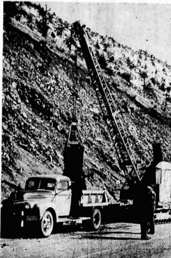
HIGHWAY DEPARTMENT MEN are feeling a few effects of Spring, having to clean up minor rock and dirt slides along the new Algoma cutoff of U.S. 97. Dirt and debris piled up this winter behind a retaining wall between the mountain and the road.
