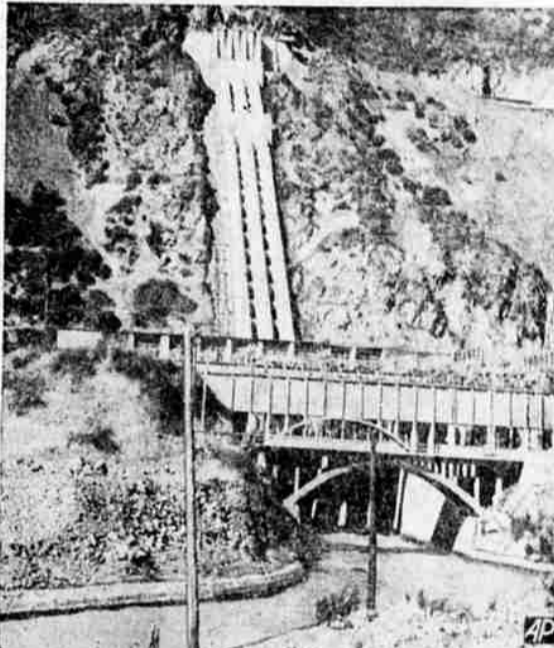
HARNESSING ANDES WATERPOWER —Water from Andes is fed by penstocks into generating station of Saual hydro-electric plant to furnish power for Santiago, Chile.
