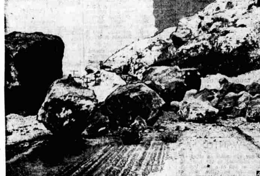
BOULDERS BLOCK HIGHWAY — Huge boulders fill U.S. Highway 30 in Echo Canyon 30 miles east of Ogden, Utah, completely blocking passage. They fell from jagged cliffs of canyon wall and stopped just short of mainline Union Pacific railroad track at left. Road crews estimated the highway could be cleared in 12 hours.
