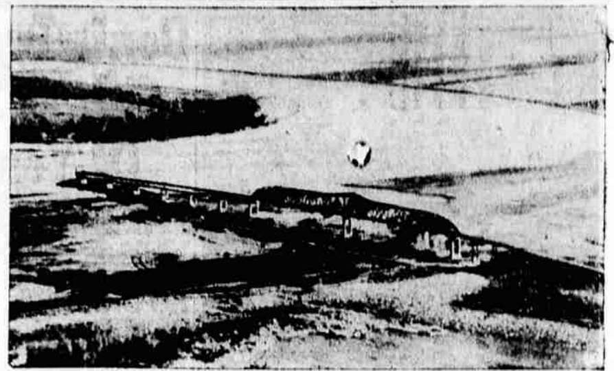
HIGH AND DRY — The meandering Missouri River played a trick on the engineers and made this $1,970,000 bridge an object of controversy. The river wandered away from the channel that was to have been crossed by the bridge between Decatur and Onawa, Ia., rendering it useless. Now, Army engineers say they have no money to steer the river back to its normal course and residents of the area are awaiting impatiently for some action toward getting the river back under the bridge.
