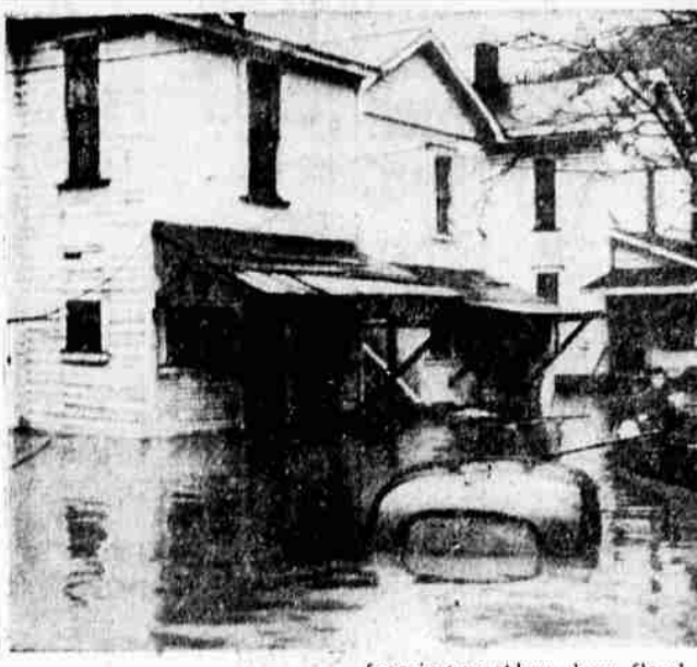
... freezing weather slows flood.
