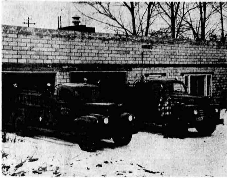
MALIN'S CITY AND RURAL fire trucks and the new fire station.
